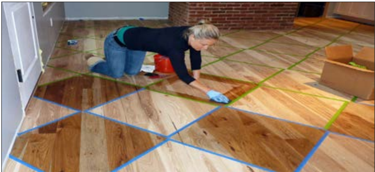
Fig 1.8.8 (v): Wood staining done by rag to create patterns (finecutwoodflooring.com)
