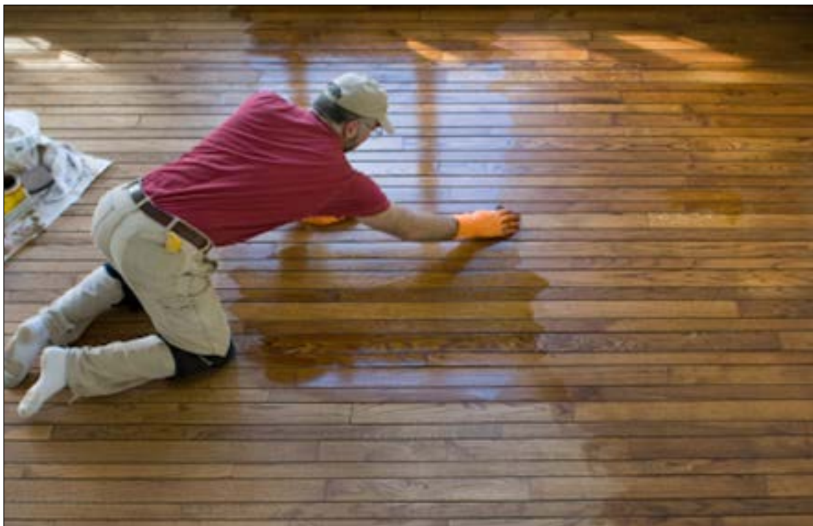
Fig 1.9: Wooden floor being polished (keylocksmithdubai.com)
