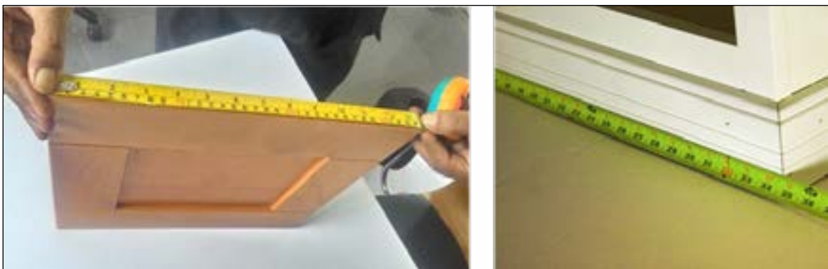
Fig 2.1.7 (vii): Lipping, mouldings and edges to be measured in length, running feet
