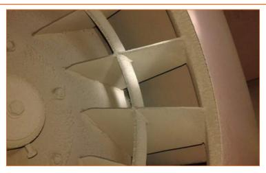
Fig 5.1.6 (iii): Dust deposits on blower to be cleaned
