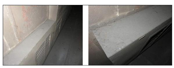
Fig 5.1.6 (i): Coating ovens found in such conditions must be cleaned
