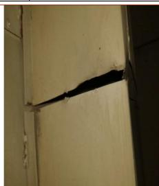
Fig 5.1.6 (iv): Oven duct conditions (damaged ducts) that must be repaired
