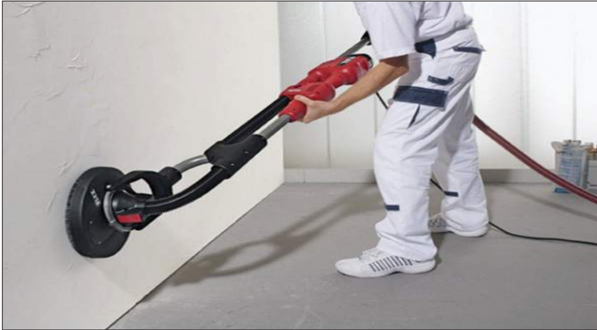
Fig 2.2 (iii): Wall sanding with electric sander (doityourself.com)
