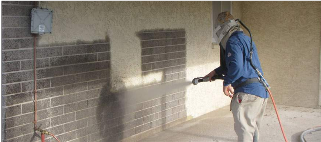
Fig 2.2.1 (ix): Sand blasting interior wall (billtonnesen.com)
