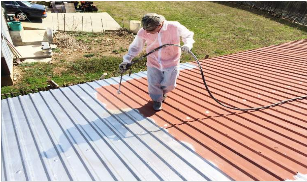
Fig 2.4 (vi): Roof being spray-painted (oldprocessroofing.com)
