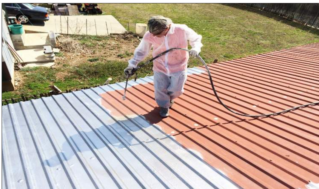
Fig 2.4 (vi): Roof being spray-painted (oldprocessroofing.com)
