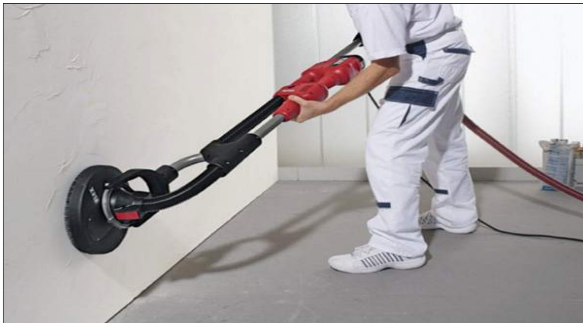
Fig 2.2 (iii): Wall sanding with electric sander (doityourself.com)
