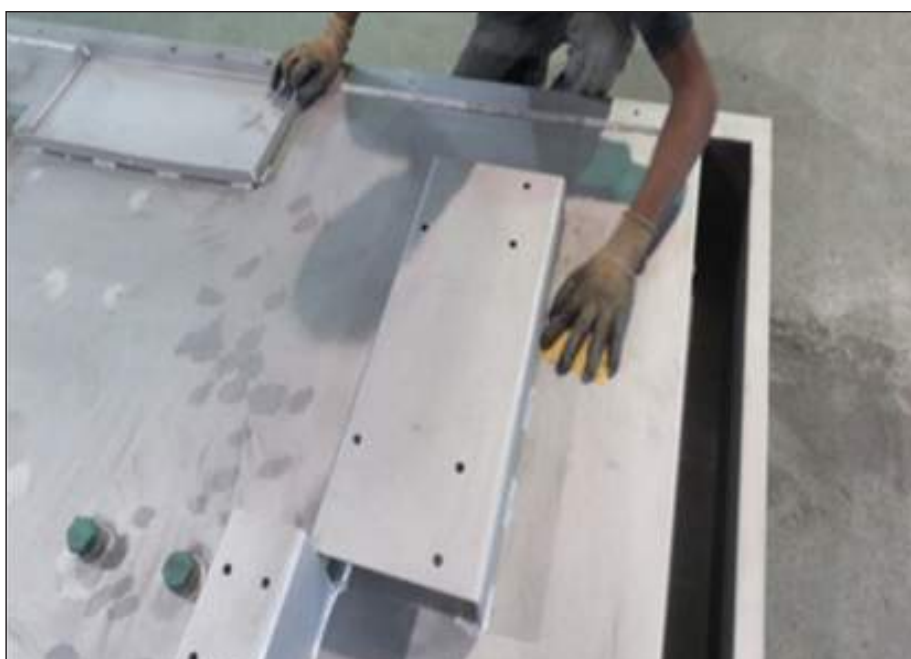
Fig 2.2.1 (iv): Hand cleaning
