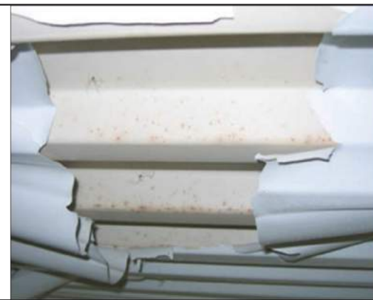
Fig 4.2.2 (x): Inter-coat delamination
