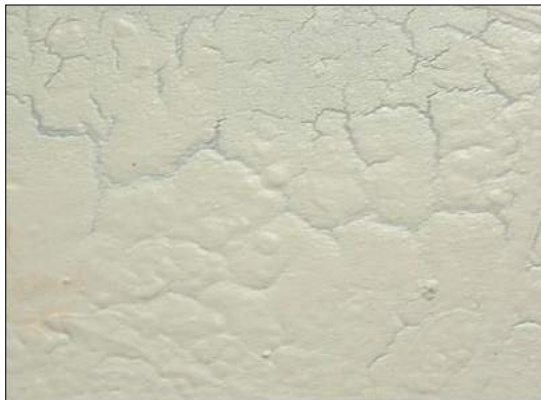
Fig 4.2.2 (vii): Mud cracking
