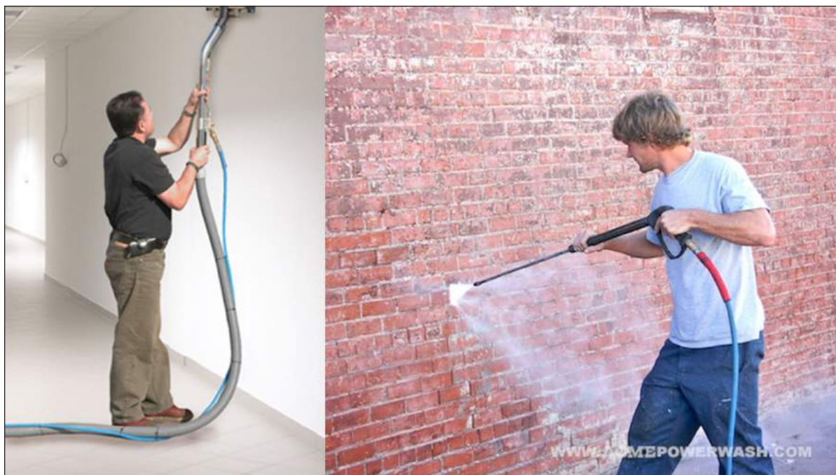
Fig 2.2 (i): Wall steam cleaning machine and pressure washing a brick wall
