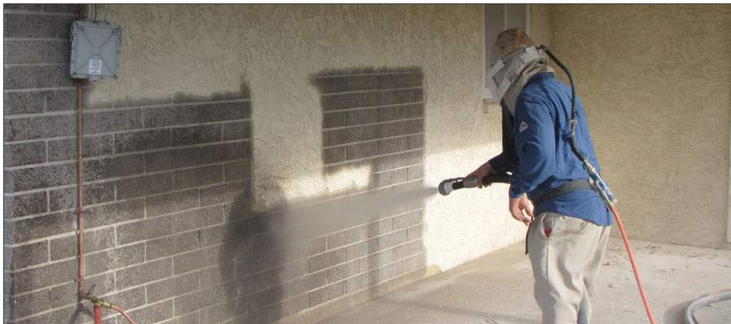
Fig 2.2.1 (ix): Sand blasting interior wall (billtonnesen.com)
