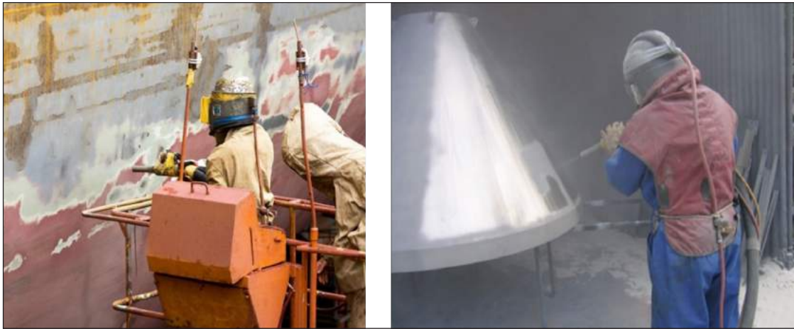
Fig 2.2.1 (x): Manual abrasive blasting
