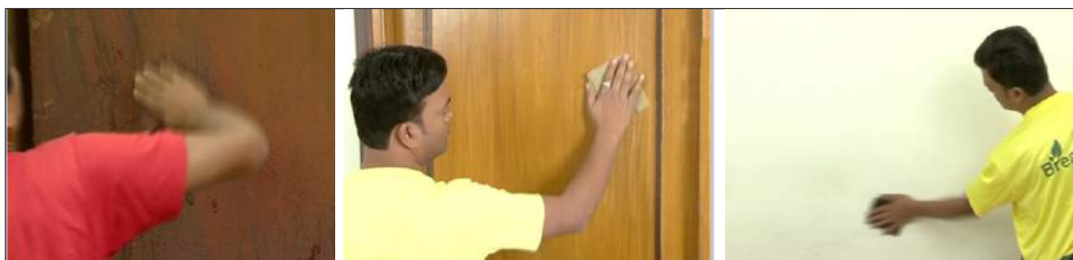
Fig 2.2 (ii): Metal, wood and wall sanding
