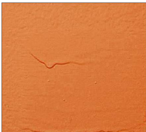
Fig 4.2.2 (i): Sagging of paint coating
