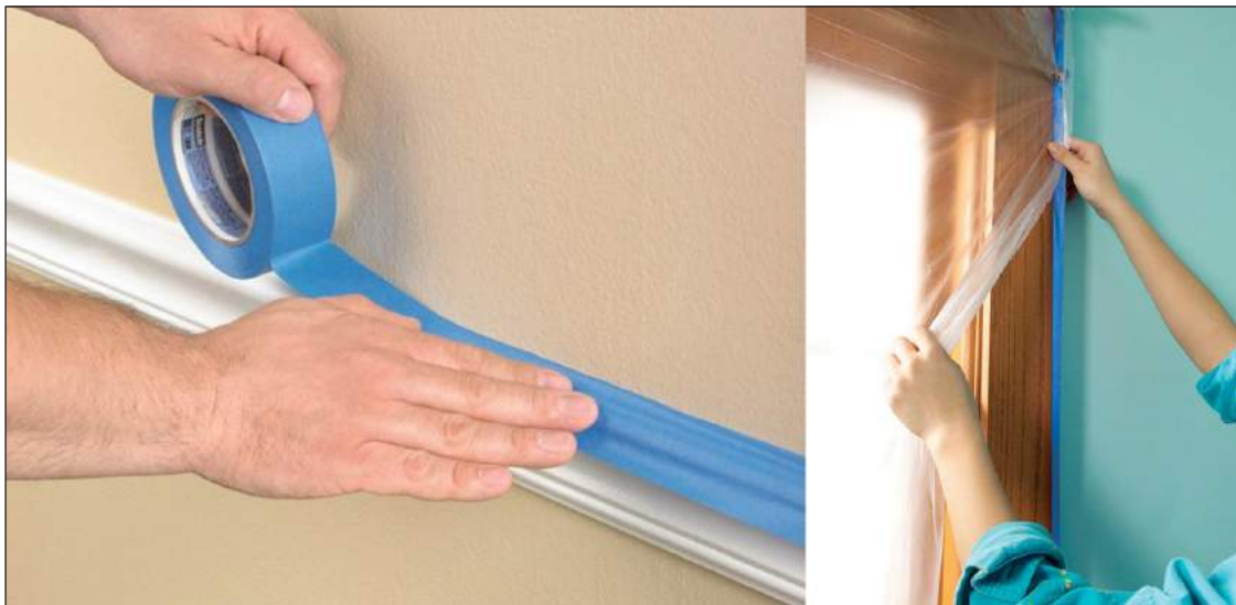
Fig 2.2.1 (xi): Masking with tape ( vancouver.sun.com and listinspired.com )
