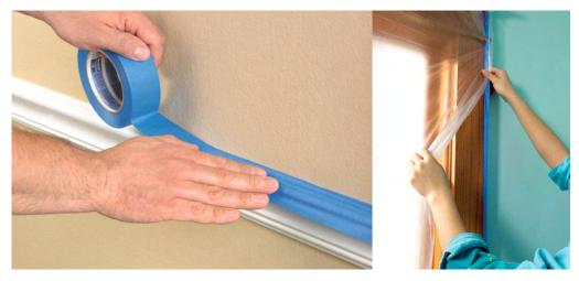
Fig 3.1 (viii) Masking with tape (vancouversun.com and listinspired.com)
