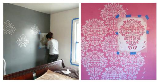
Fig 5.2 (iii) Stencilling (diybydesign.blogspot.in, techillin.com)
