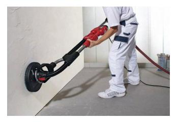
Fig 4.1 (ii): Wall sanding with electric sander (doityourself.com)
