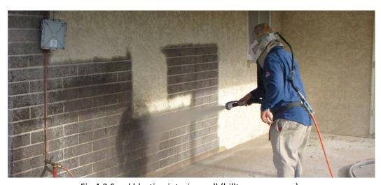
Fig 4.3 Sand blasting interior wall (billtonnesen.com)
