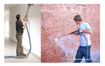
Fig 4.1 (i) Wall steam cleaning machine and pressure washing a brick wall
