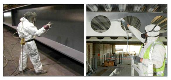
Fig 4.5 (vi) Airless spray technique
