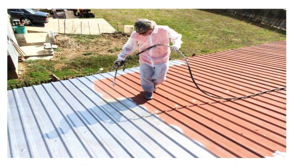
Fig 4.5 (I) Roof being Spray-Painted (oldprocessroofing.com)
