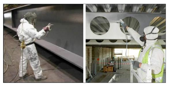
Fig 2.4 (xi): Airless spray technique
