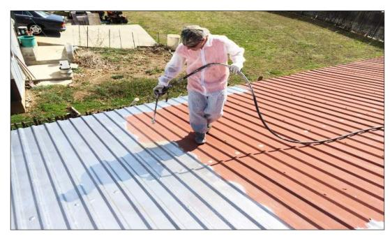
Fig 2.4 (vi): Roof being spray-painted (oldprocessroofing.com)
