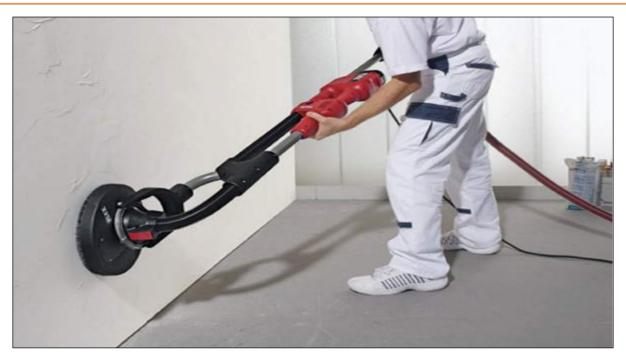
Fig 2.2 (iii): Wall sanding with electric sander (doityourself.com)
