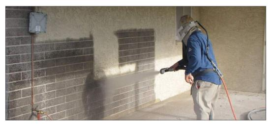
Fig 2.2.1 (ix): Sand blasting interior wall (billtonnesen.com)
