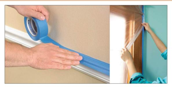
Fig 2.2.1 (xi): Masking with tape (vancouversun.com and listinspired.com)
